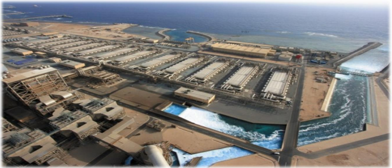
<Desalination Plant at Jeddah, KSA>
